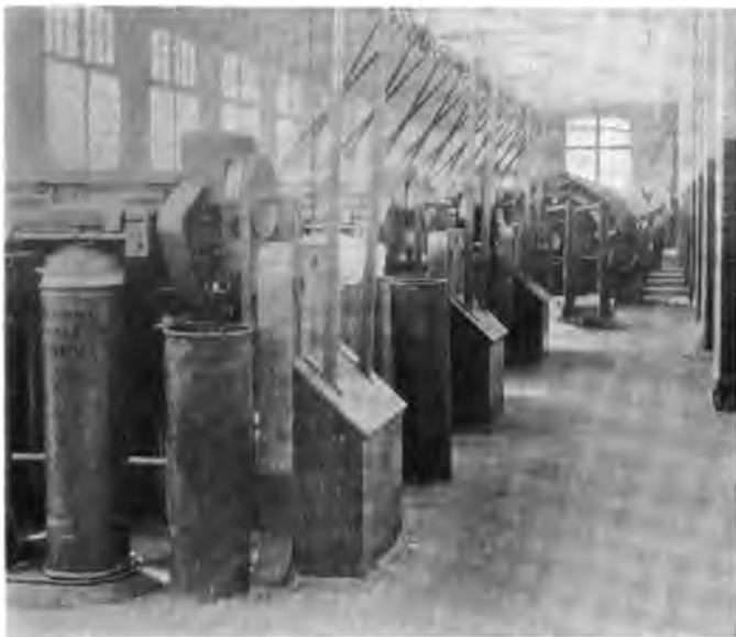
Fig. 2. Belt Guards for Drawing Frames.
